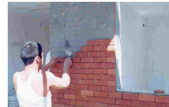
Fig. 7: Enchape de ladrillo
