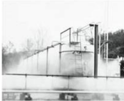
FIGURE 16.9.1 Water Spray Protection for LP-Gas Tanks
